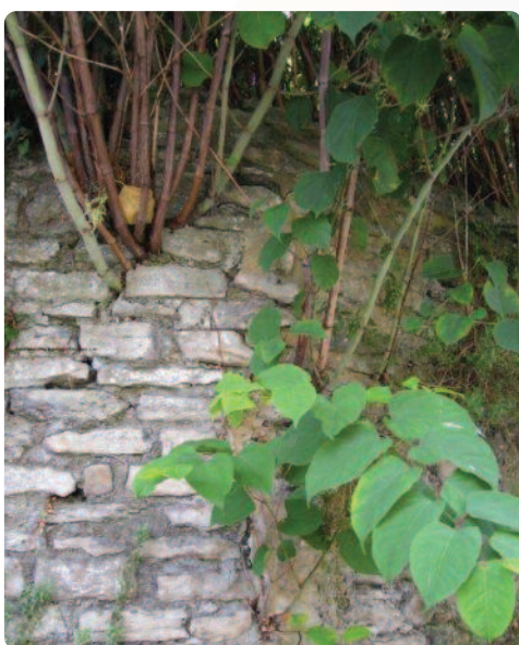
Photos showing Knotweed growing through boundary walls
