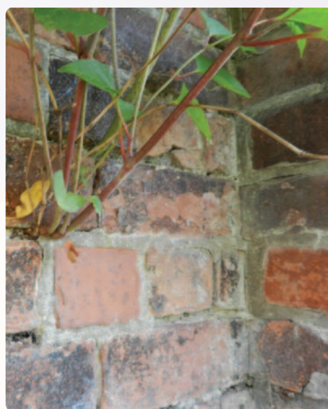
Photos showing Knotweed growing through boundary walls
