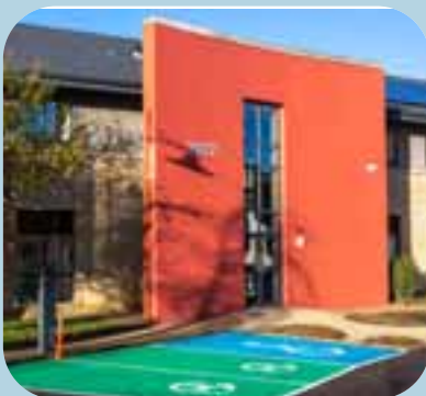
Upgraded building entrance, with new landscaping and EV charging points.
