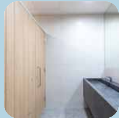
Upgraded WC facilities with water reduction taps.
