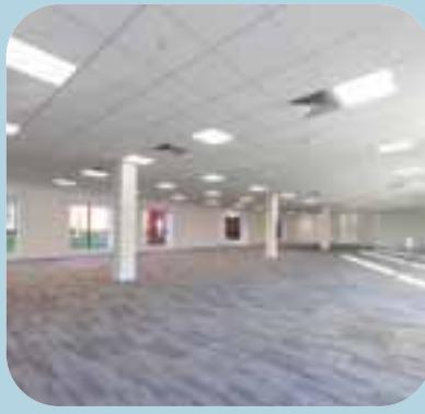
Upgraded office space with LED daylight sensor lighting.
