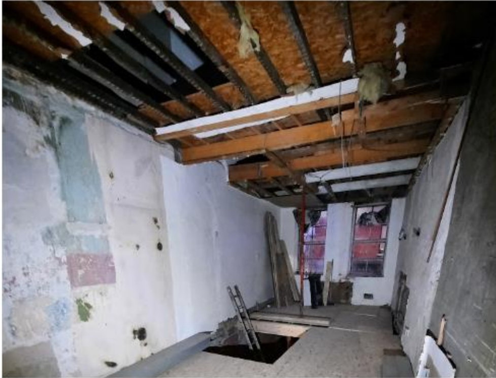
Replacing of floors on a vacant building. Appropriate contingency allowed for on the project.
