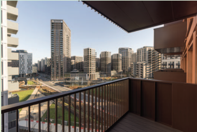
The innovative clip-on balcony system was manufactured offsite and installed using a co-ordinated crane strategy, reducing onsite welding, hot works and temporary edge protection requirements.
