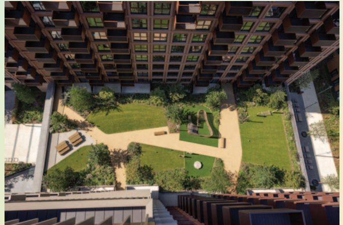
Precast concrete façade panels eliminated the 'double carbon' effect of traditional brick over concrete façades, and delivered substantial savings.
